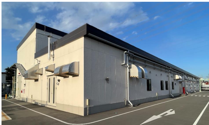
A-SOLiD™ is produced in this mass production testing building.
